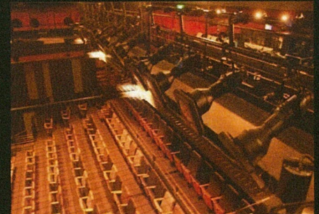
Tension Wire Grid
